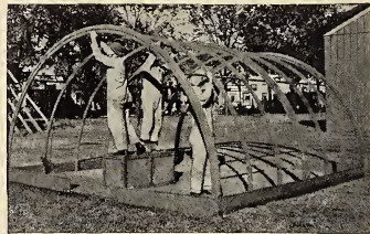
The shelter going up.
